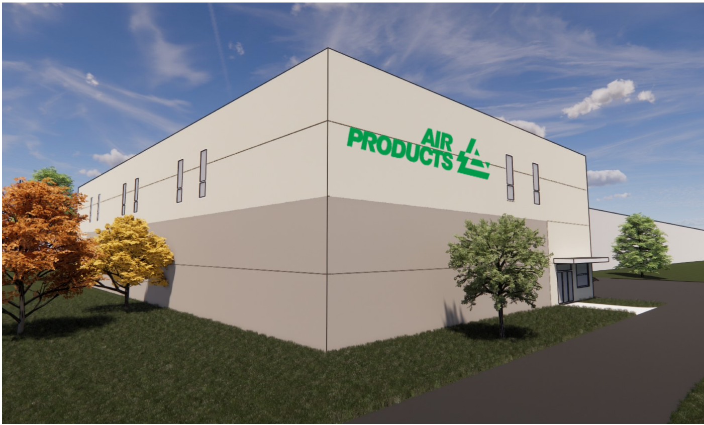
WAREHOUSE BUILDING NORTH/WEST VIEW
